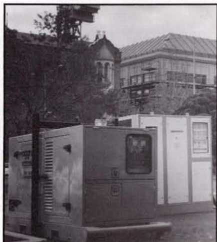
Canopied "Hushpower" 60kva Generator and Load Bank.
